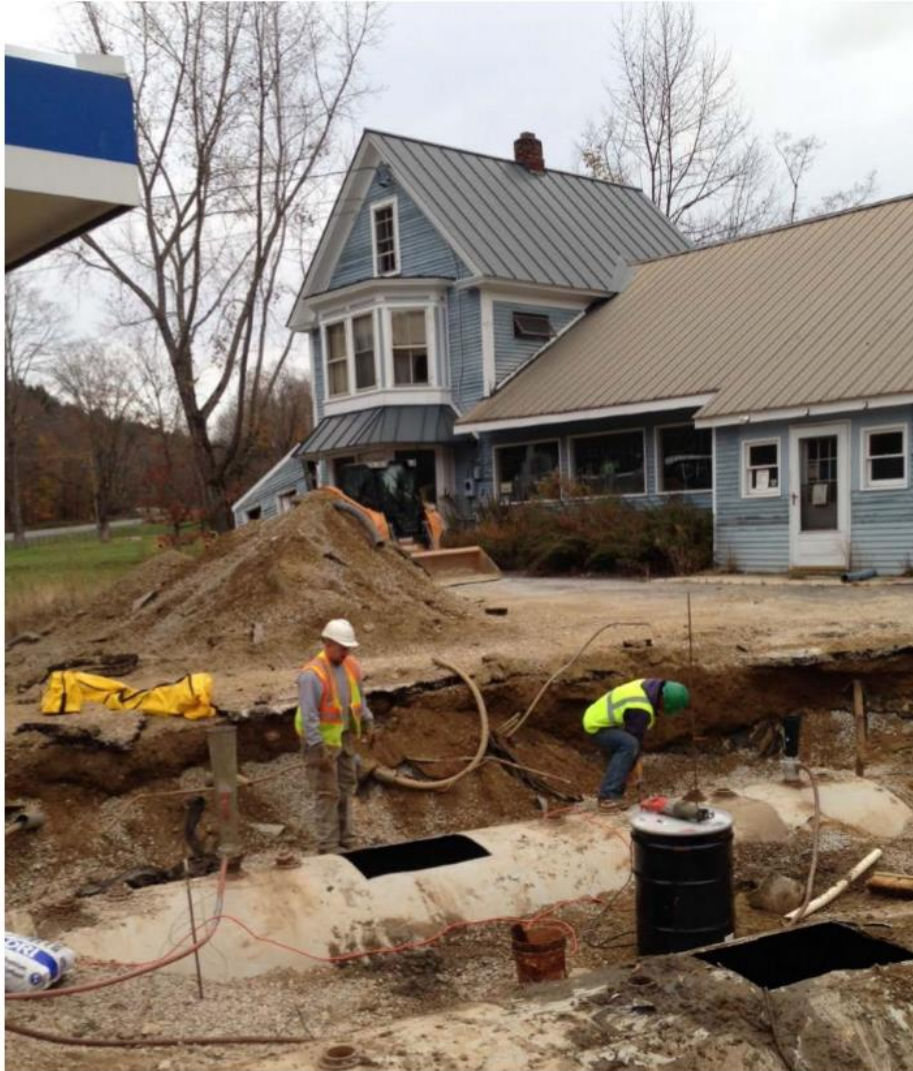
Removal of fuel tanks as part of site assessment and cleanup and site with erosion control going into place on final grade.
